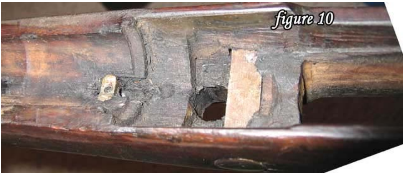
Close up of barrel channel and recoil lug area. Again, it's nice and clean, these are some of the hardest areas to degrease on a rifle.
